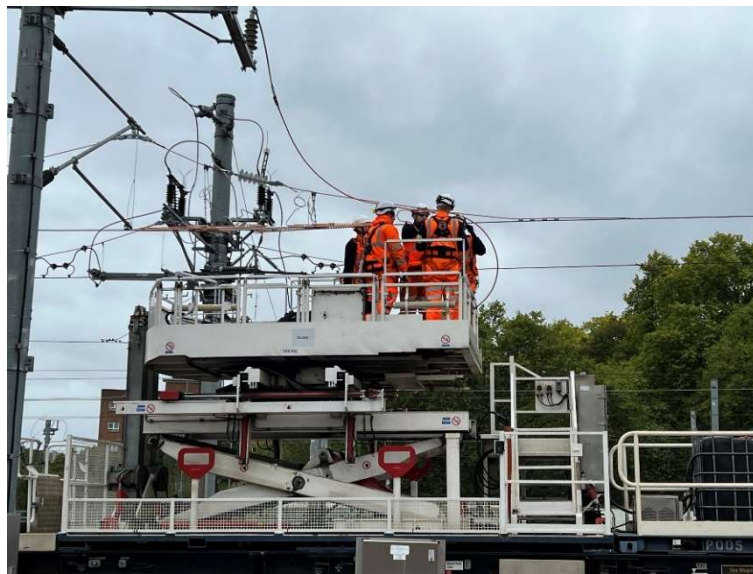
FIGURE 19 - SECTION INSULATOR WORKS BEING COMPLETED AT ST PANCRAS
