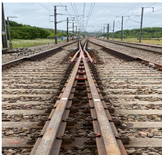
FIGURE 22 - 2242 SWING NOSE CROSSING, NASHENDEN
