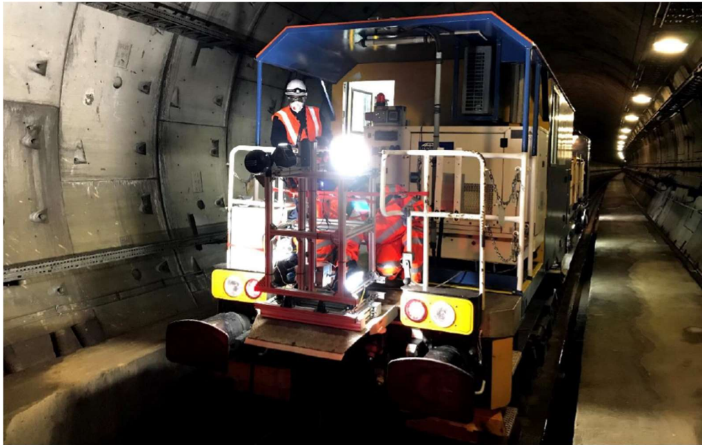
FIGURE 10 - THE MPV WITH THE TUNNEL VISION EQUIPMENT INSTALLED RECORDING TUNNEL CONDITION
