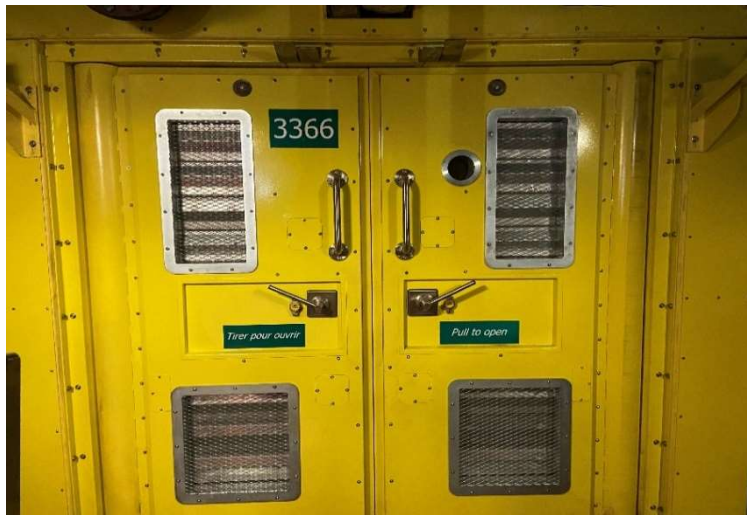
FIGURE 20 - COMPLETED CROSS PASSAGE DOOR RENEWALS IN THAMES TUNNEL
